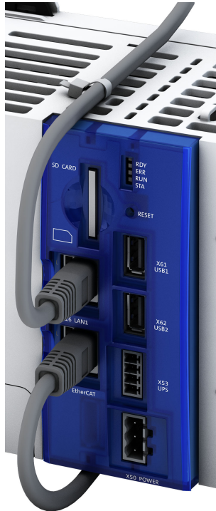
Fig. 2: Installation and fixing of the network cables
